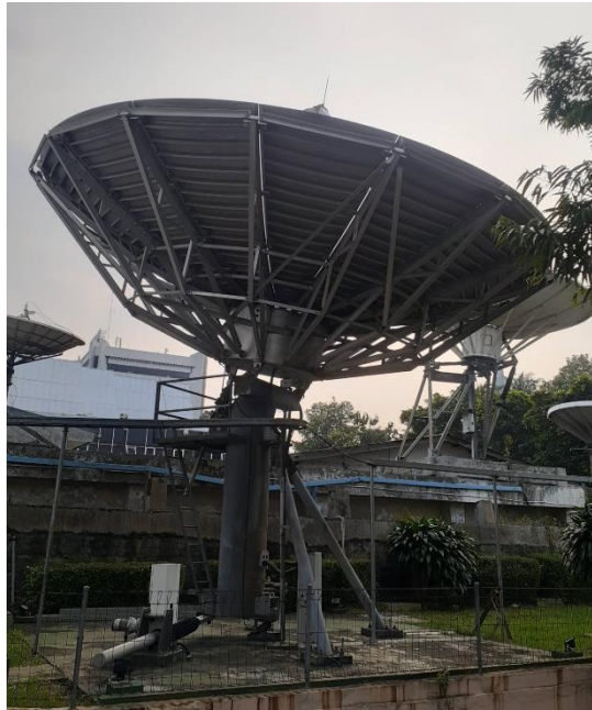
Gambar 3.2 Antena Parabola LPP TVRI
