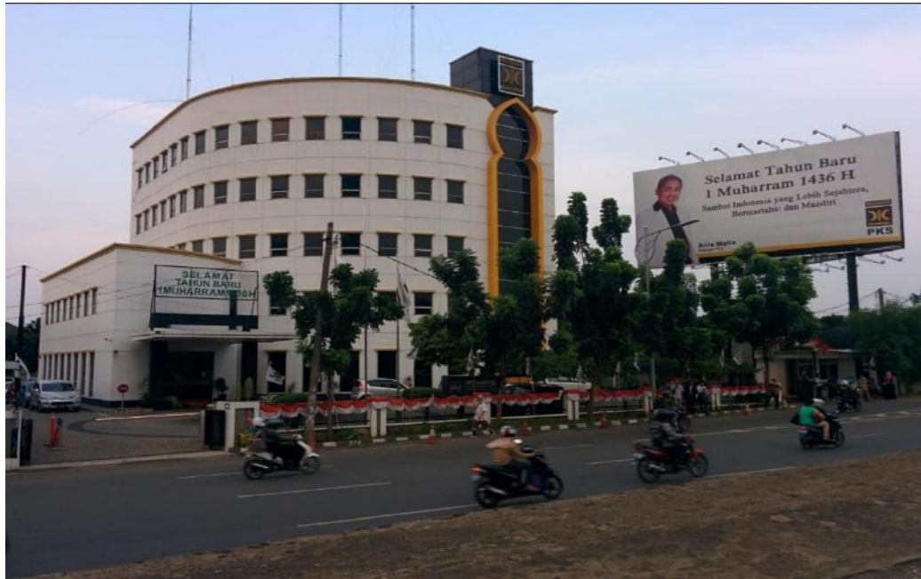
Figure 1 The dakwah centre or Markaz Dakwah (MD) of DPP-PKS, Jakarta
