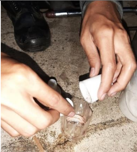
Figure 5. The Process of Mixing Resin and Catalyst
