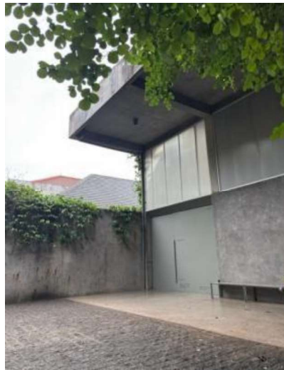
Figure 1: Roh Projects Art Gallery at Cikini front view
