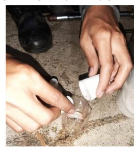
Figure 7. The process of mixing resin and catalyst
